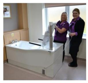
approved Showersafe gantry system which prevents the backflow of the contaminated water to Category 5 level and an auto fill system that fills the bath to a pre-determined maximum limit as well as a digital temperature
